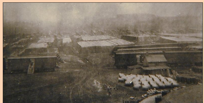
Above: This grainy AC&Y construction image shows ground loading of sewer pipe at an unknown location, likely either Robinson Clay in East Akron or Colonial Brick in Mogadore. Note ramps were utilized allowing sewer pipe to be pulled into boxcars. ( ACYHS Archive )
