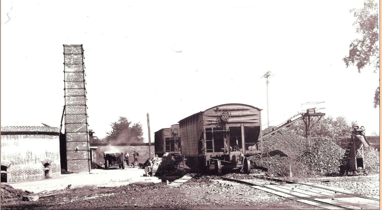
TWO RAILROAD COAL HOPPERS AT THE UNLOADING DOCK AT THE E. BIGLOW CO. IN NEW LONDON, OHIO IN 1950. THE SMALL CART IS FULL OF HOT CINDERS FROM ONE OF THE KILNS.
