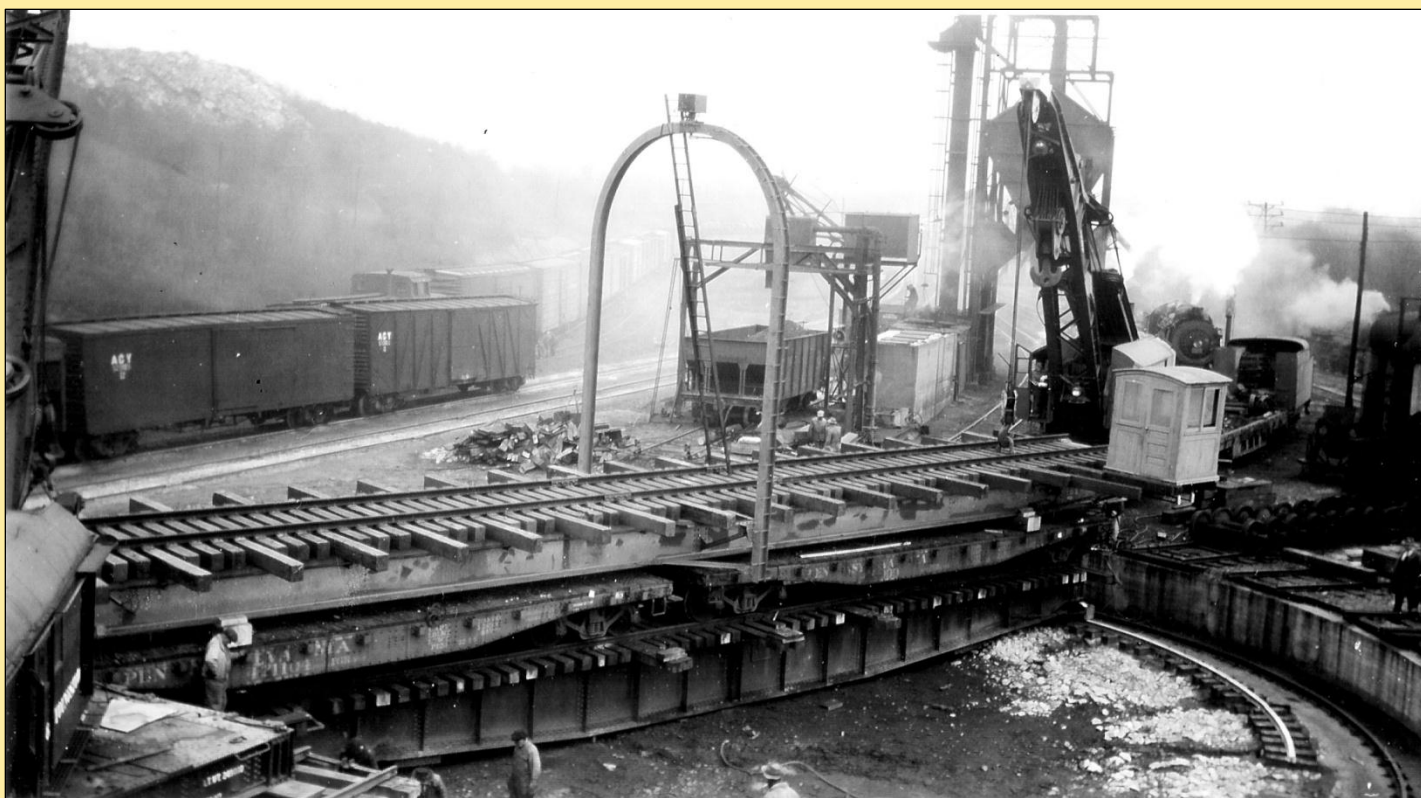
Above: This image shows several details worthy of comment. First, the installation of the new 90-foot turntable at Brittain in late 1946 required deployments of both AC&Y X-991 steam derrick and a steam crane rented from the W&LE. Next, both the original steam ash hoist and new Ross & White conveyor are visible beyond the turntable arch. The circa 1921 hoist may have been retained pending assured flawless operation of the new electric ash conveyor. Lastly, just left of the arch is the only known image of the first AC&Y Stores car number 4. AC&Y HS Archive.
