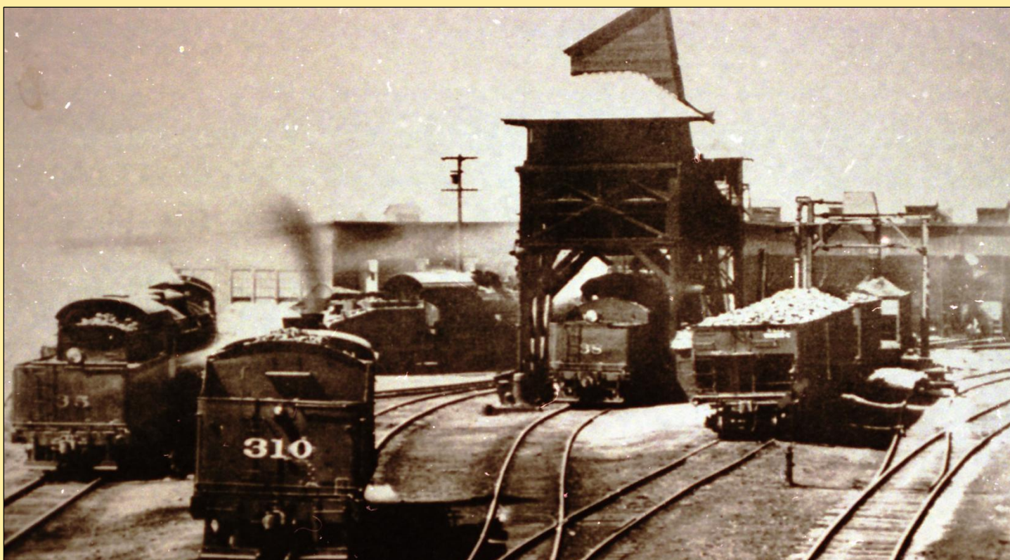
Above: The busy AC&Y Brittain terminal as it appeared in 1925 with the original steam ash hoist. AC&Y HS Archive.
