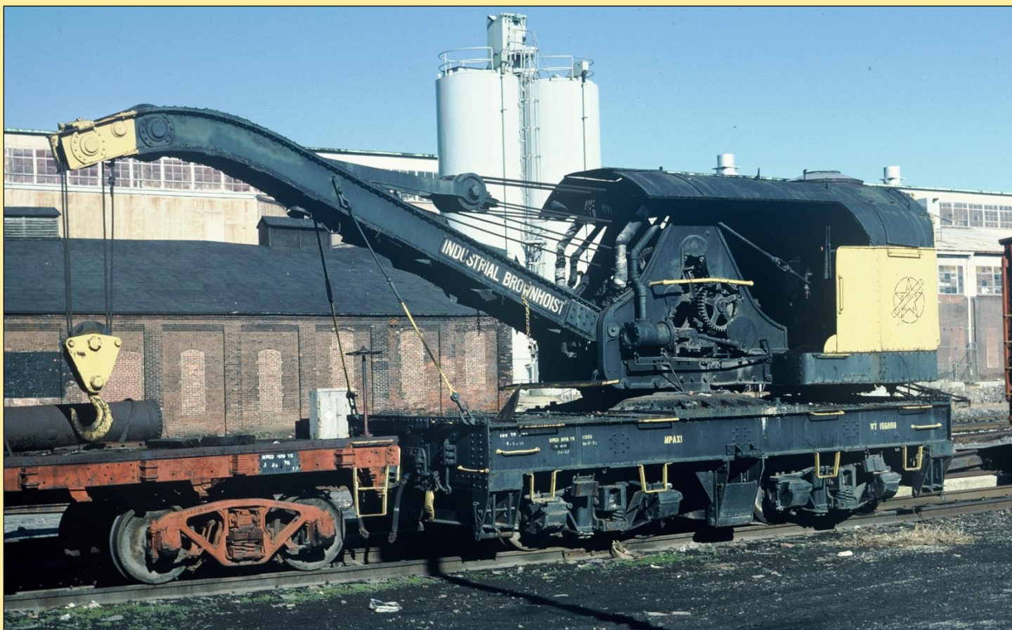
Above: Though out-of-service, Emons era MPA (Maryland & Pennsylvania) X-1 is seen in July 1986 at York, PA. Then 87-years young, the old steam wreck derrick unfortunately did not survive the scrapper's torch despite valiant efforts to find a new home. Reportedly, the former AC&Y X-990 was too heavy to be moved over poor roads. Alan Mende
