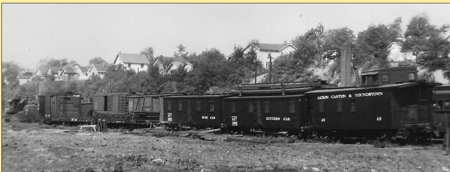
Above: At same location at Brittain is the wreck relief outfit in July 1946 with caboose 40. Also in view is tie car X-989, extra gang rail flat X-988, tool car X-983, derrick X-991 with idler X-987. It is believed the tie and rail cars were assigned to the MOW Dept., not usually in the standing wreck relief outfit. C. W. Burns, Society Archive collection.
