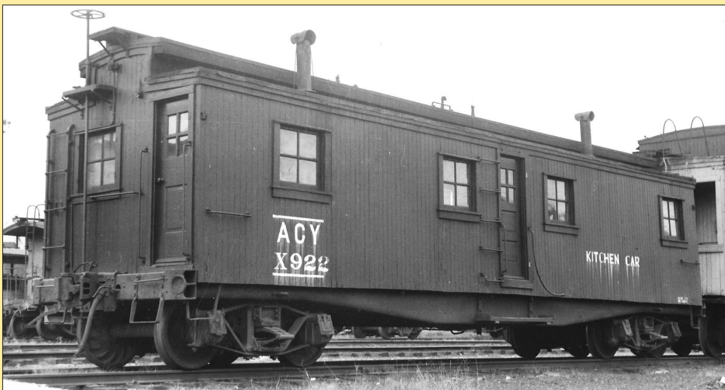
Above: A former Pennsy boxcar was converted in 1926 to AC&Y's relief wreck X-922 kitchen diner car. The X-922 appears respectively at Brittain in 1953 and 1952. Retirement came in 1966. Bill Nixon collection, Bob's Photo.
