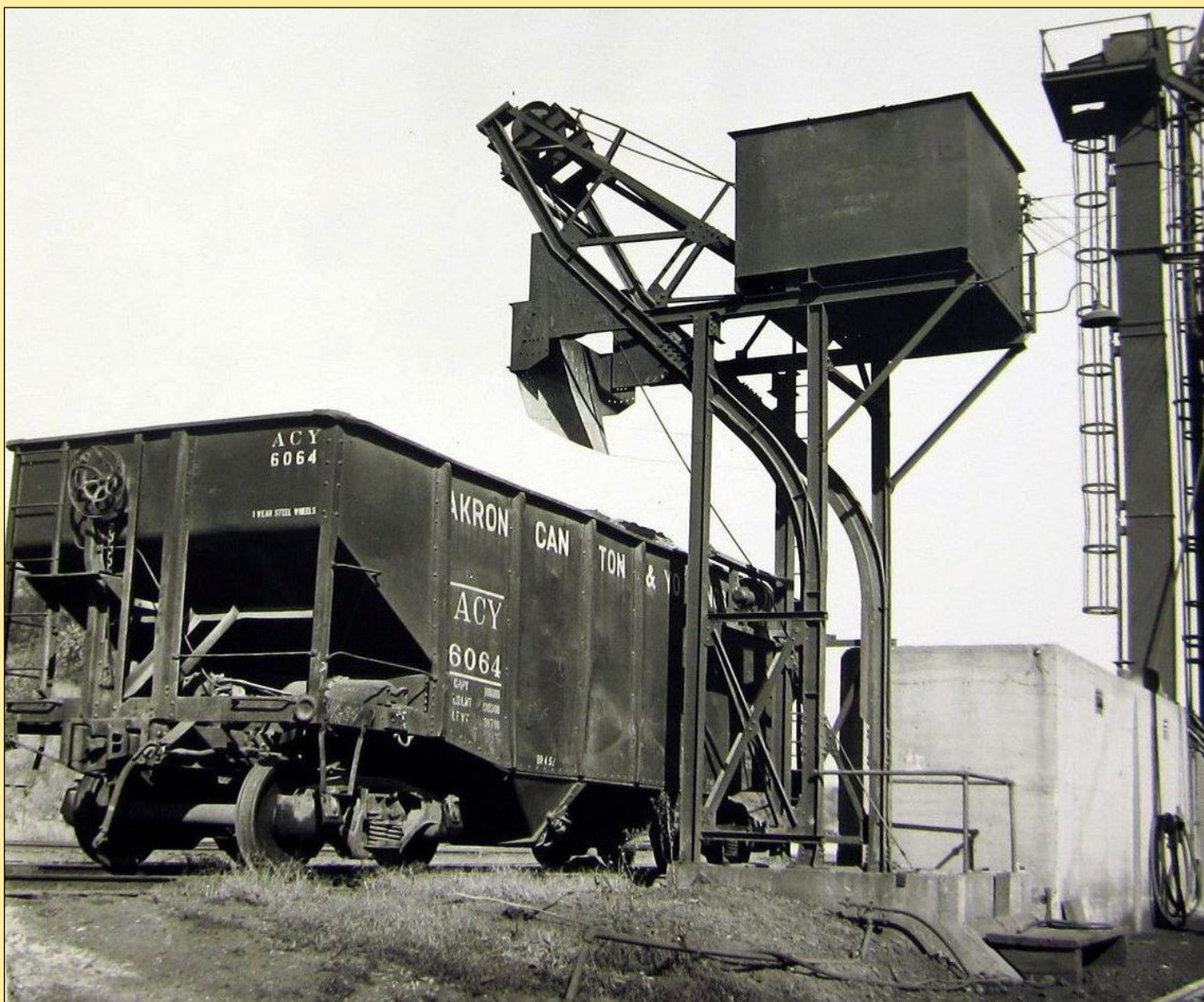
Above: The Ross & White ash hoist / cinder conveyor is featured at AC&Y's Brittain terminal. Bob Lucas collection.
