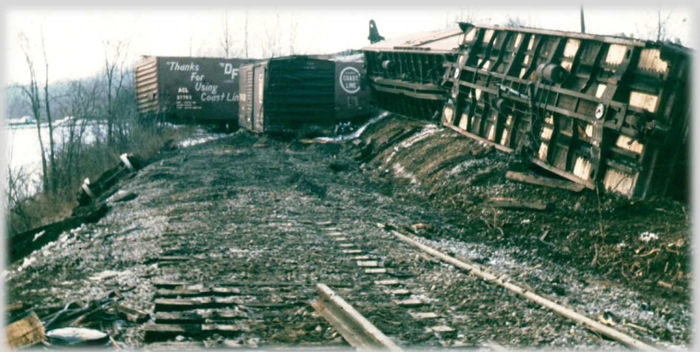
Above: Another later view of the 1966 Tymochtee derailment shows the right-of-way. The track was likely removed to allow bull dozers to clear damaged equipment so the line could be reopened. Note the new wood floor showing on the overturned boxcar to the right. Jim Robert' photo, author's collection.
